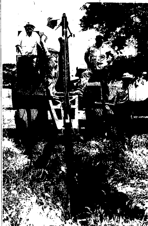
BARBECUE PIT FOR 2,500 pounds of choice beef is being dug here by, left to right, Bill Pfeil, Al Bahe, Mel Reeg and Hans Rath-wich, in preparation for the Thursday night barbecue. See story at right for details.
